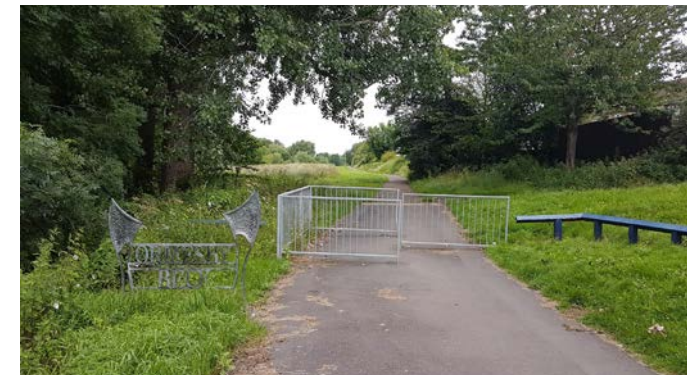
▲ Entrances to walking and cycling routes can act as barriers to wheelchair users than others when not thoughtfully designed.
