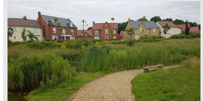
▲ A SuDS installation included as part of Middlesbrough’s recent Grey Towers Village development.
