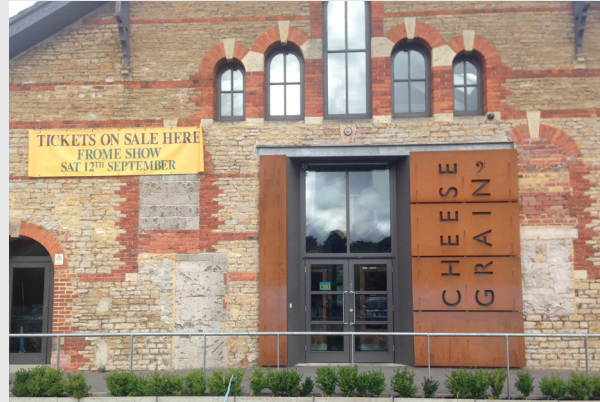
The restored market hall in Frome because a focal point in the town's wider regeneration agenda, and is managed by the community
